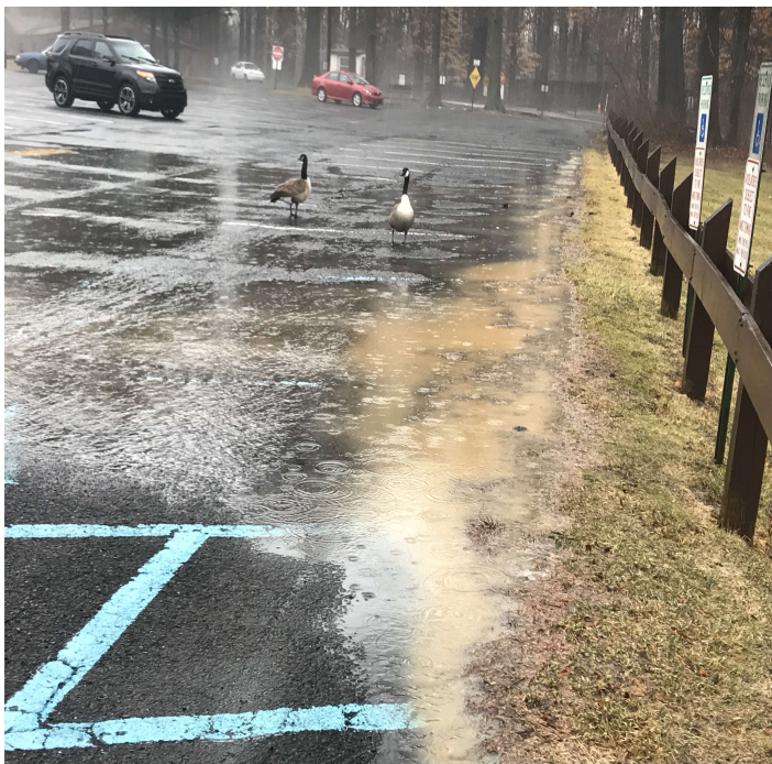
Photos: (left) Parking lot is pitched towards Forrest Ave. (right) Drainage is conveyed through an eroded channel.
