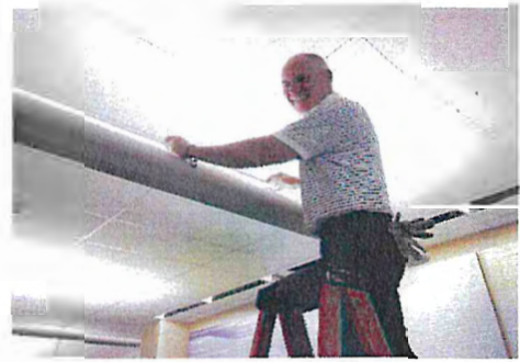
Bill Griffenburg installing LED lighting
