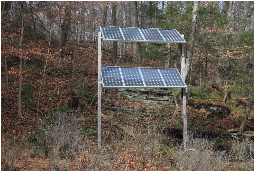
Solar Energy System, Ground-Mounted
