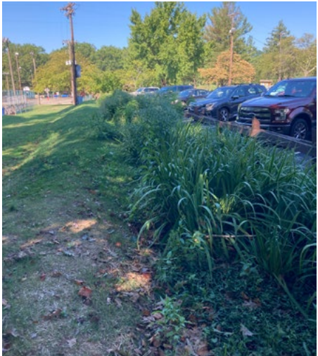
▲ New infiltration swale at Alverthorpe Park
