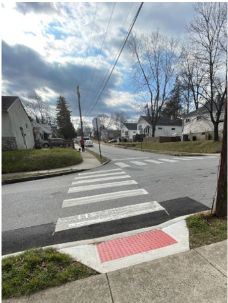
▲ Photo example of an ADA curb cut and detectable warning surface at Ardsley Park
