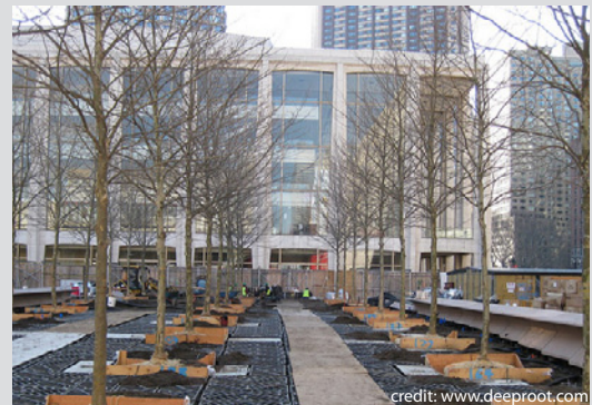
Fig. 2.4.29 - Precedent of Silva Cell construction
