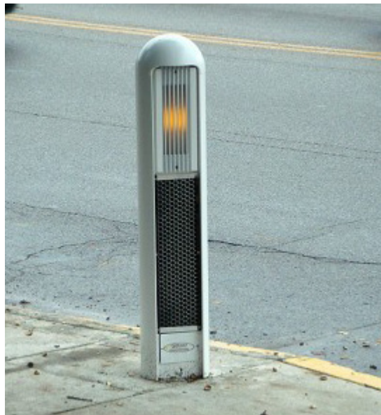
Figure 18: Bollard with sensor that activates flashing lights only when a pedestrian is waiting to cross.
