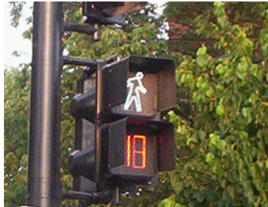
Figure 11: Countdown crossing signals that display the time remaining for safe crossing.
