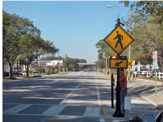
Figure 17: Flashing pedestrian signal with LED lights to alert drivers when a pedestrian is trying to cross.
